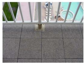
After all full tiles are installed make the necessary cuts around obstructions. The last row of tiles toward the bldg. may need to be cut in order to fit. Leave a 1/4" gap around the outside perimeter of the covered area for expansion and contraction.
