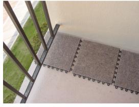
Suggested starting point is the outside edge with a full tile the loops towards the face of the bldg, and the opposite side of the deck
